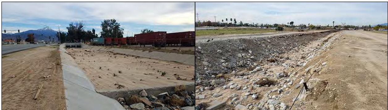
Figure 4. Current conditions of the City Creek Channel. Left : concrete-lined channel near Victoria Avenue, view to the east; right : earthen channel in the middle portion, view to the west. (Photographs taken on December 10, 2019)
